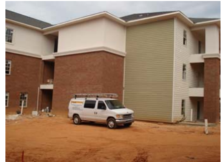
Exterior painting and work on pool begins
