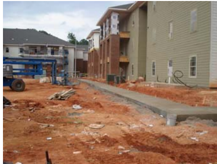
Sidewalks and Parking Lot Underway
